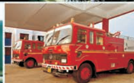
Fully functional fire station
